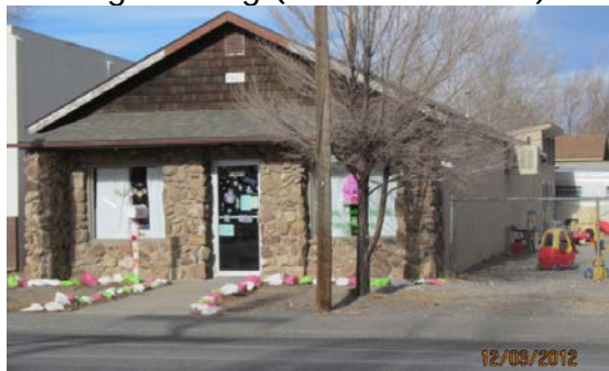
Existing Building (Addition at back):
